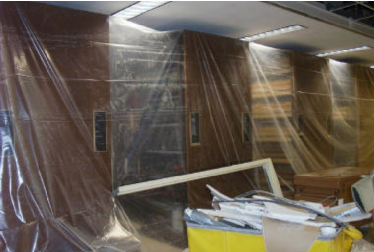
More construction to break down the training room.
